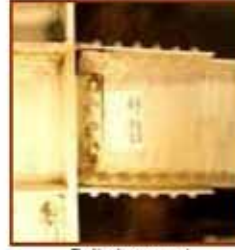
Bolted moment connection
